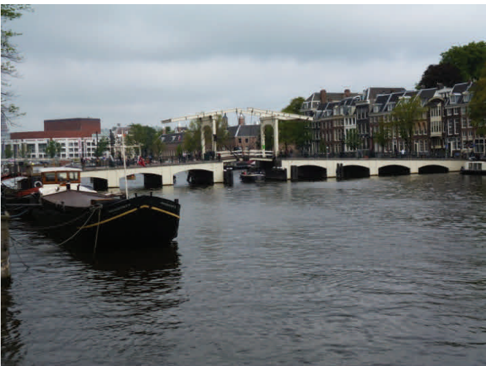
Figure 8 Amstel Bridge, Amsterdam, NL
